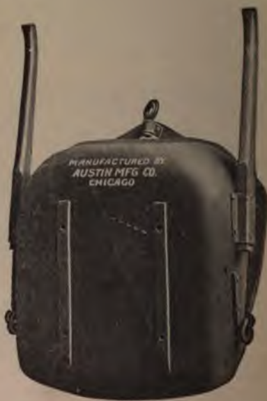
Rear View of Drag Scraper with Runners.
